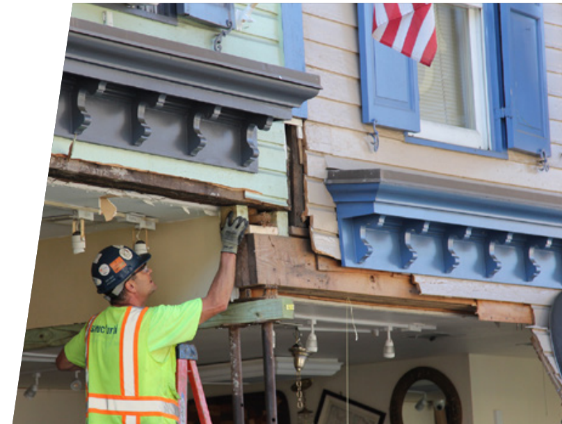
Building stabilization after severe flood damage in Ellicott City, Maryland. PHOTO BY PRESERVATION MARYLAND
